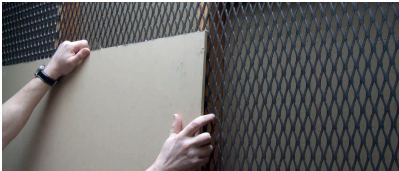
High security plasterboard installation
